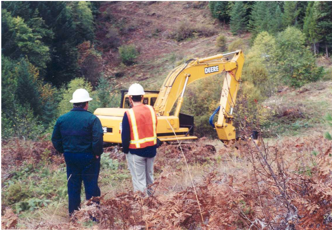
Figure 6.1. Right-of-way reclamation using mechanical control. In this case, a slashbuster.
