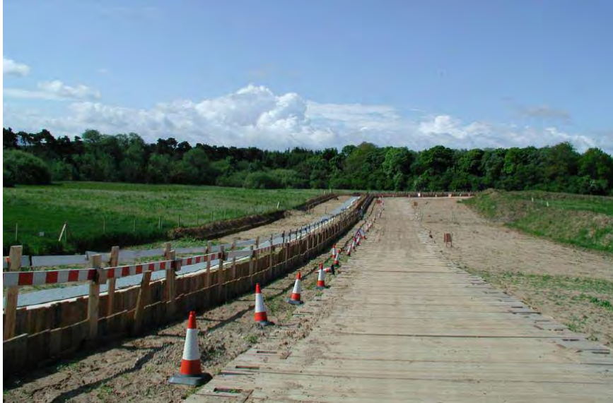
Figure BB-3. Typical Cable Construction ROW with Single Cable Trench Open
