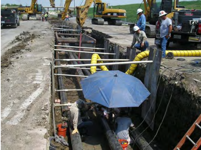
Figure BB-1. Typical HPFF Pipe Installation
