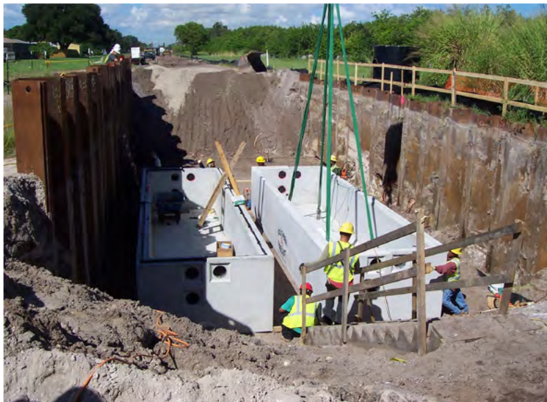
Figure BB-4. Typical XLPE Vault Installation
