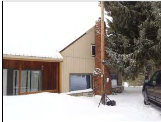
17 18 Photograph taken in the direction of the primary residential structure
