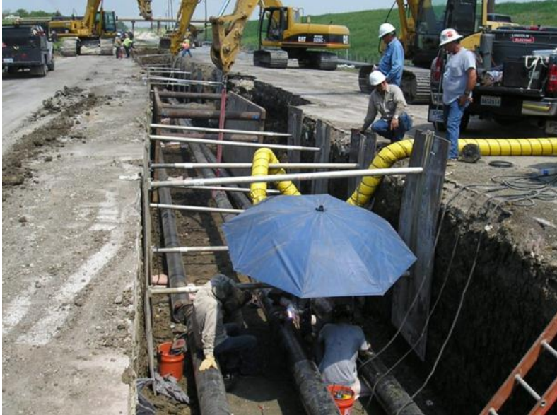
Figure BB-3-1. Typical HPFF Pipe Installation
