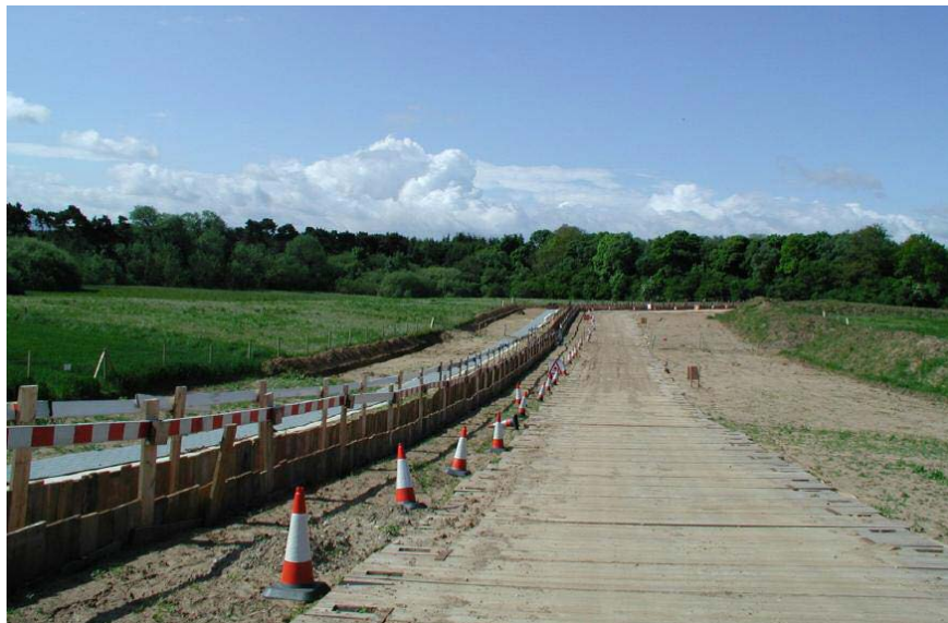
Figure BB-3-3. Typical Cable Construction ROW with Single Cable Trench Open
