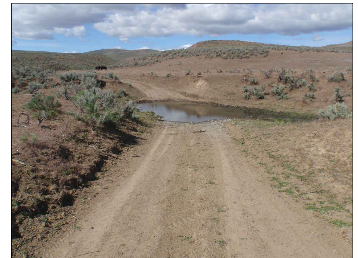
SITE PHOTO - FACING NORTH (MAY '14)
